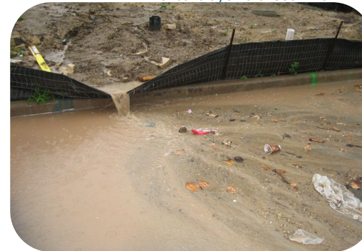
Damaged or ineffective BMPs
